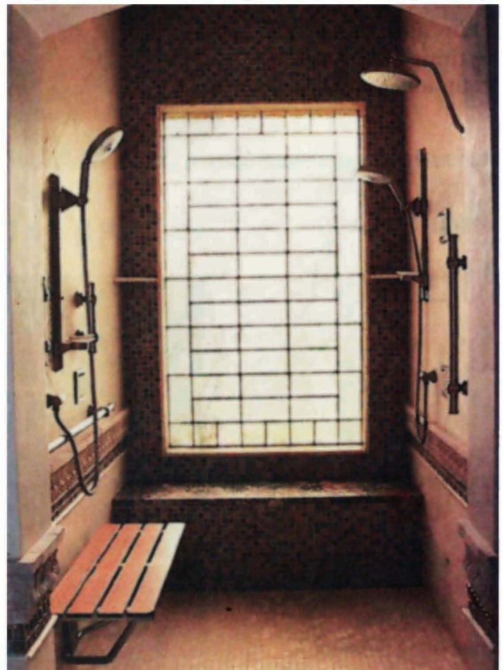
This sumptuous shower has been designed to allow users to stand or sit in comfort. It could also easily accommodate a wheelchair user.
