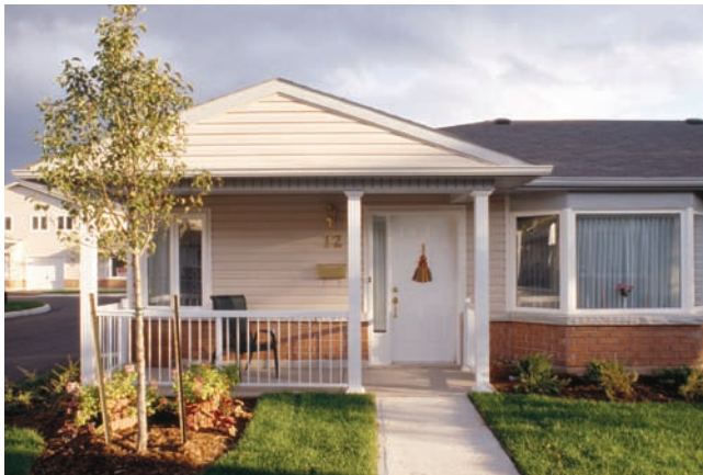
At Woodside Mews, a life-lease community for the elderly in Oakville, Ont., houses have design features such as at-grade entries that allow seniors to age in place.
